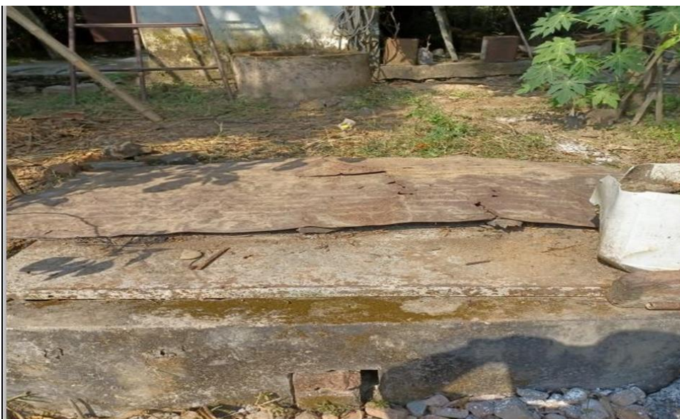
Unnamed Road, Himachal Pradesh 176206, India
